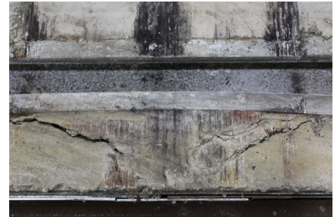
Cracks on concrete surface due to frictional forces
