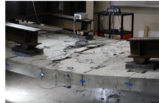
Localized concrete crushing
